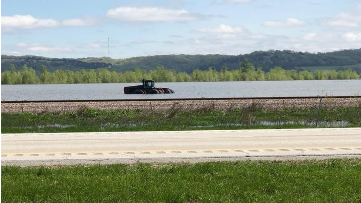
Figure 4. Floodwaters Adjacent to Roadway (Photo Credit Dr. Scott Schram, Iowa DOT)
